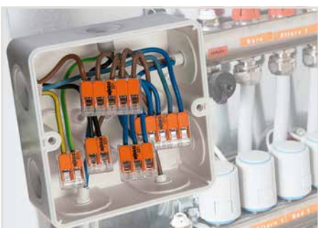
Wiring fine-stranded conductors in a junction box.
