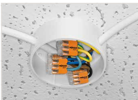
Lighting distribution in ceiling canopy
